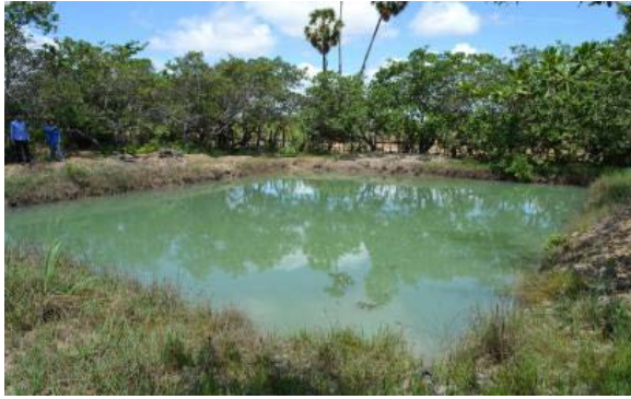
Retention ponds (Source: WOCAT, T_CBD005en)
