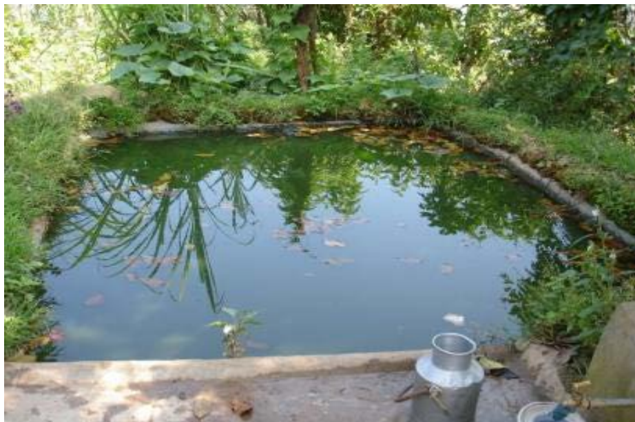
Plastic-lined detention ponds (Source: WOCAT, T_NEP022en)
